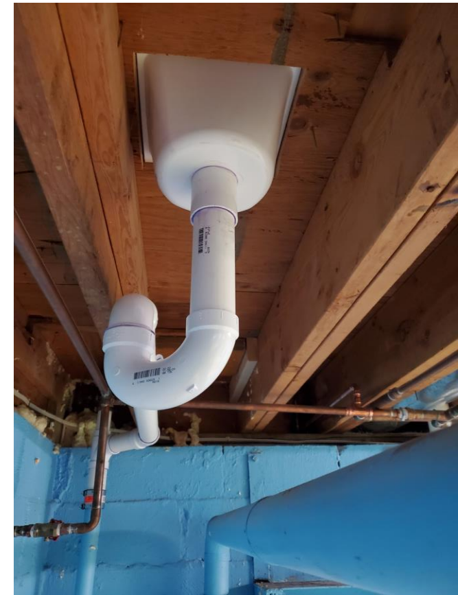
Drain located under the outlet of the bath
