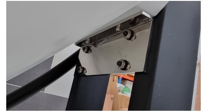
Stainless steel brackets attached To black powder coat steel frame
