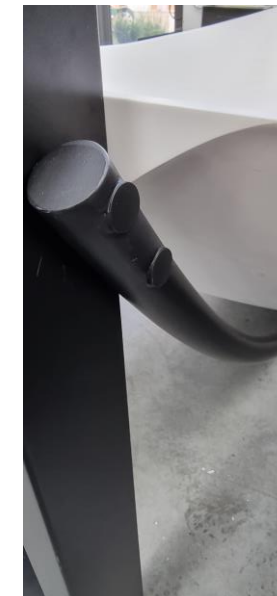
Curved brace connected to steel frame
