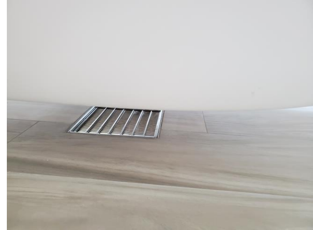
Drain located under the outlet of the bath
